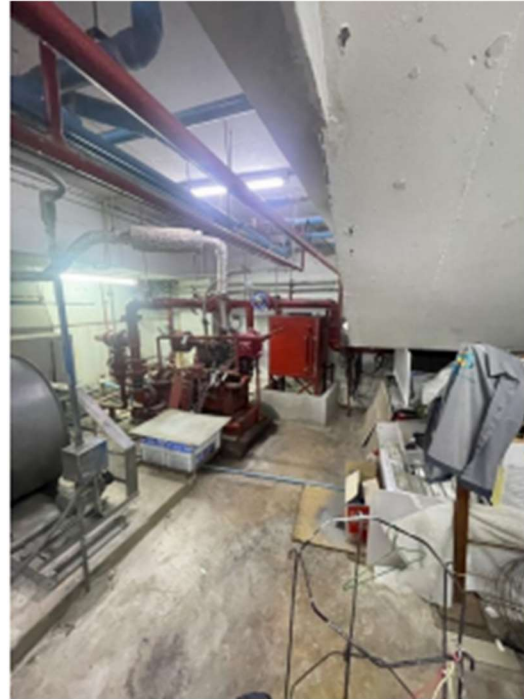
Water pump and fire pump on underground floor
